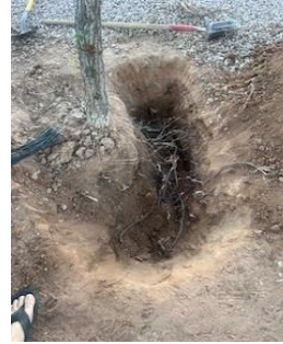
Tree roots took out Communication wire at #5 CW
