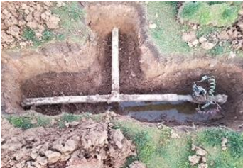
Irrigation repairs at CW during April
